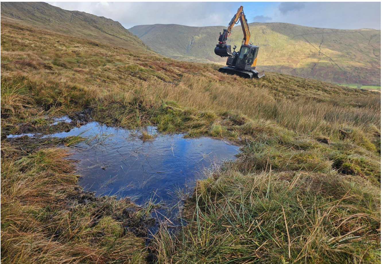
A digger working behind a pool created by a bund.
