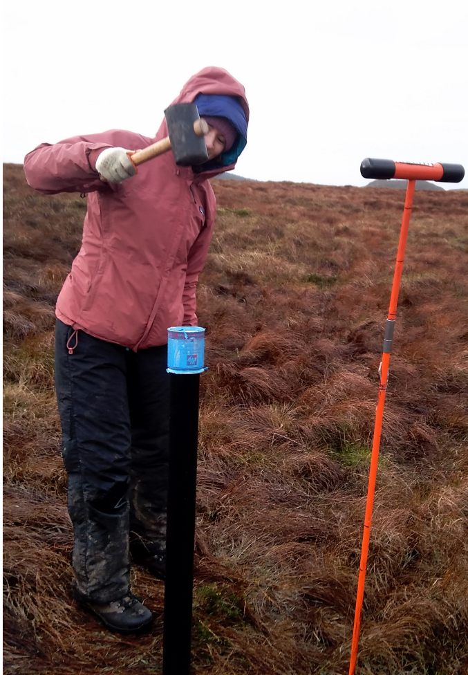
Above - a volunteer installing a dipwell
